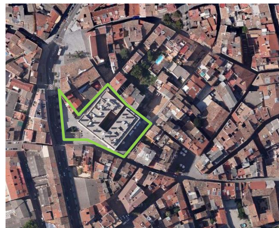
Figure 10. Current state of target urban area: Quatre Cantons, Manresa
